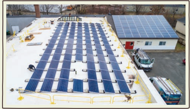
New 31 kW solar array on our flat roof! (Photo: Jerry Monkman Photography)
